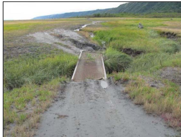
One of the bridge crossings at the fingers of Wallace Creek in the Fox River Critical Habitat Area. By relocating the bridge to higher, drier ground there should be reduced impact by ORV use. Part of this project includes a revegetation plan to ensure the re-establishment of native grasses.
