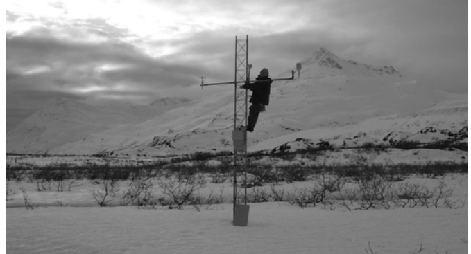
Maintenance of a SNOTEL site at Bradley Lake
