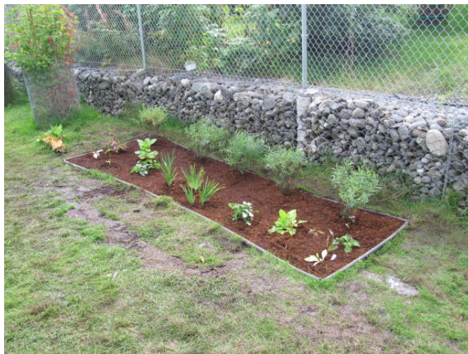
Demonstration rain garden installed by HSWCD – Aug, 2011
