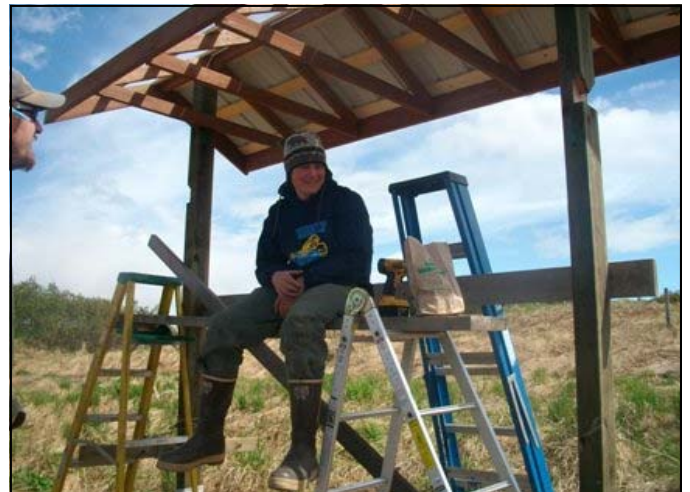
Jake McLean takes a bit of a rest during the installation of his kiosk in the Snomads parking lot at the trailhead of the Watermelon Trail. Jake organized a sizable work party to install this mammoth informational kiosk
